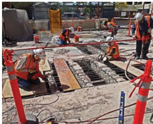
Removal of concrete topping in front parking lot
