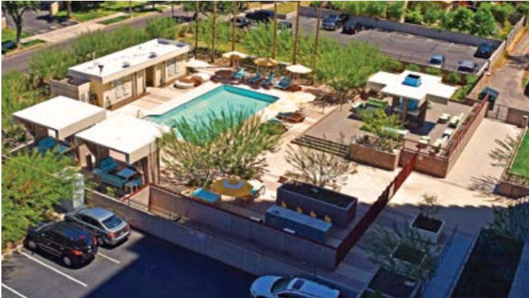
Back patio plaza area after renovation
